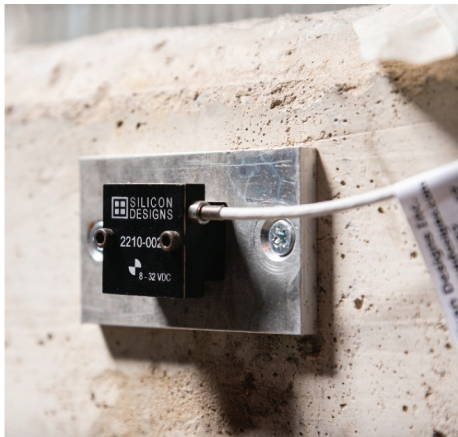
a) View of installed accelerometer sensor
