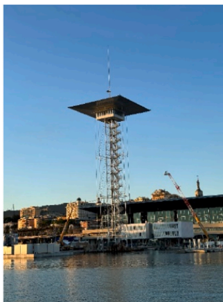
(a) Photograph of the Control Tower
